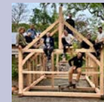
Timber frame building
